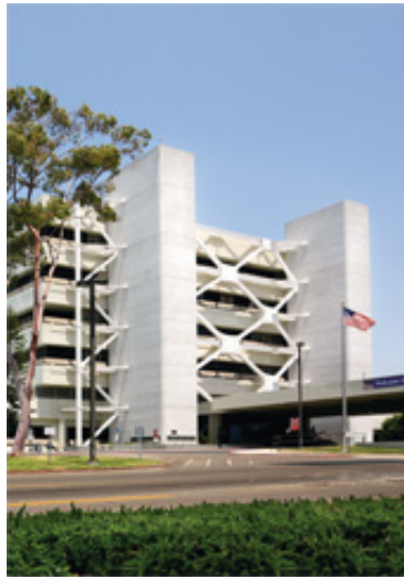
The Veterans Affairs Medical Center in San Diego was later encased in a 60 million dollar steel construction designed to stabilise the building during earthquakes.
